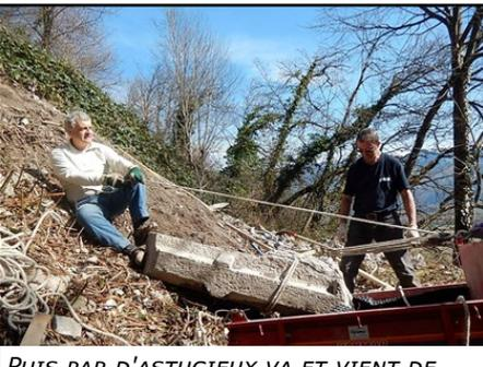
**PUIS PAR D'ASTUCIEUX VA ET VIENT DE CHENILLETTE, ET UN MOUFLE BIEN UTILE, IL FINIT PAR PRENDRE PLACE DANS LA BENNE, BIEN TROP CHARGÉE POUR LA CAUSE.**
